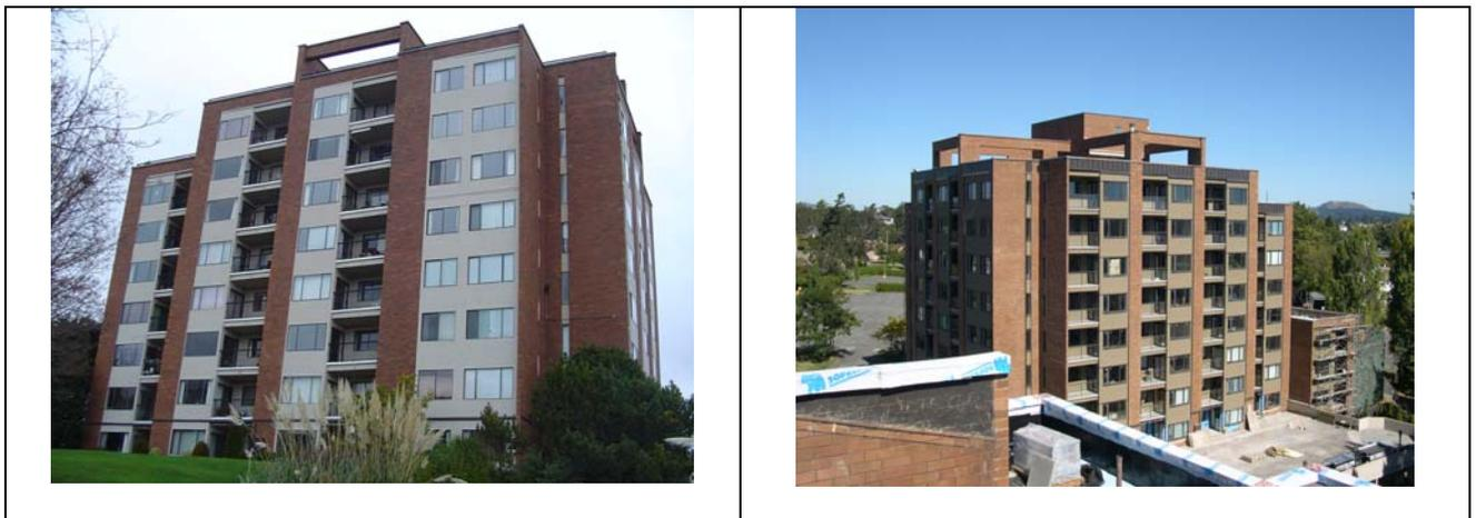
**Figure # 1:** Elevation view of unclad reinforced clay masonry wall and infill stucco façade. The photo at left has the original face seal stucco panels and the photo at right has rain screen stucco with flashing over-cladding around the perimeter of the stucco panels. The masonry was re-pointed and sealed but remained unclad. There were typically more than a dozen interfaces on each level of each façade.
