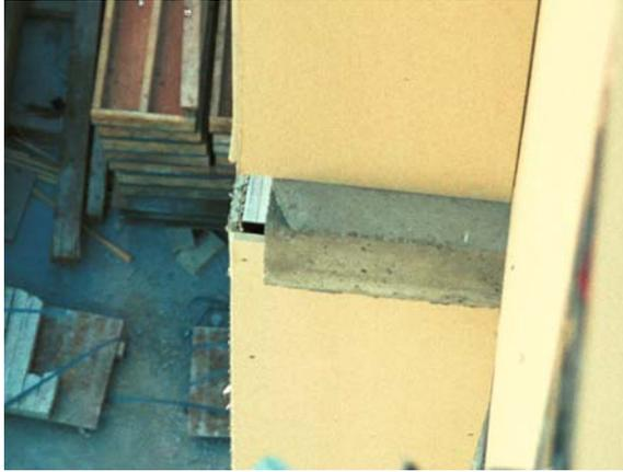
*Illustration 1: Walls and supporting slab misaligned; on one side the slab projects from the wall sheathing, on the other it's retracted. The same detail applies to both—the designer envisioned the slab edge and face of sheathing in alignment.*
