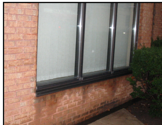
Figure 2. Flashing/wall interface
