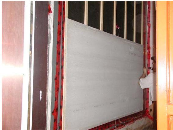
**Figure 14 - Installation of cement board (Location 7)**
