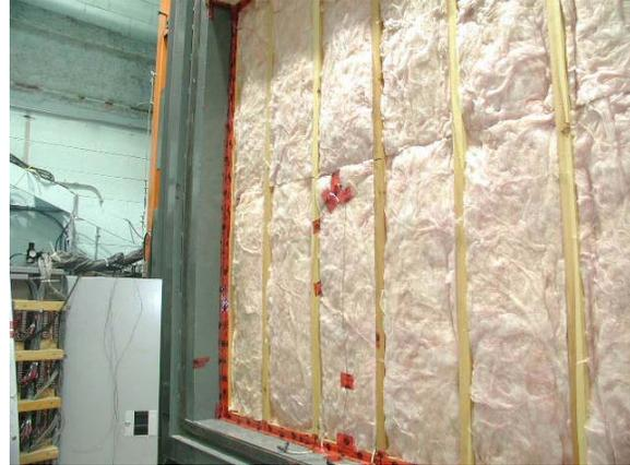
**Figure 15 - Installation of insulation in stud-cavity**
