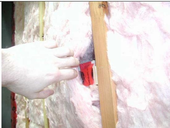
**Figure 20 - Installation of ACR sensor in stud cavity**
