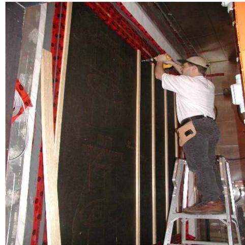
**Figure 11 - Installation of strapping for cavity behind cladding**
