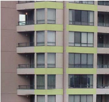
Figure 9. Stucco covered concrete upstands (denoted by light-green highlight).
