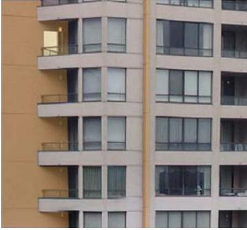
Figure 7. Painted concrete shearwalls and shearwall ends (denoted by orange highlight).
