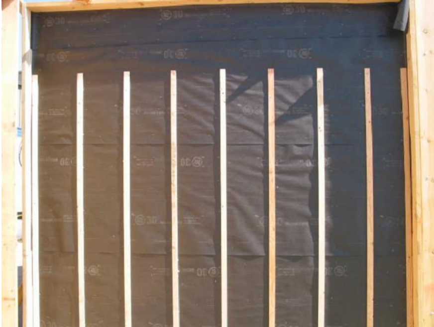
Photograph #1 – Test panel with strapping applied
