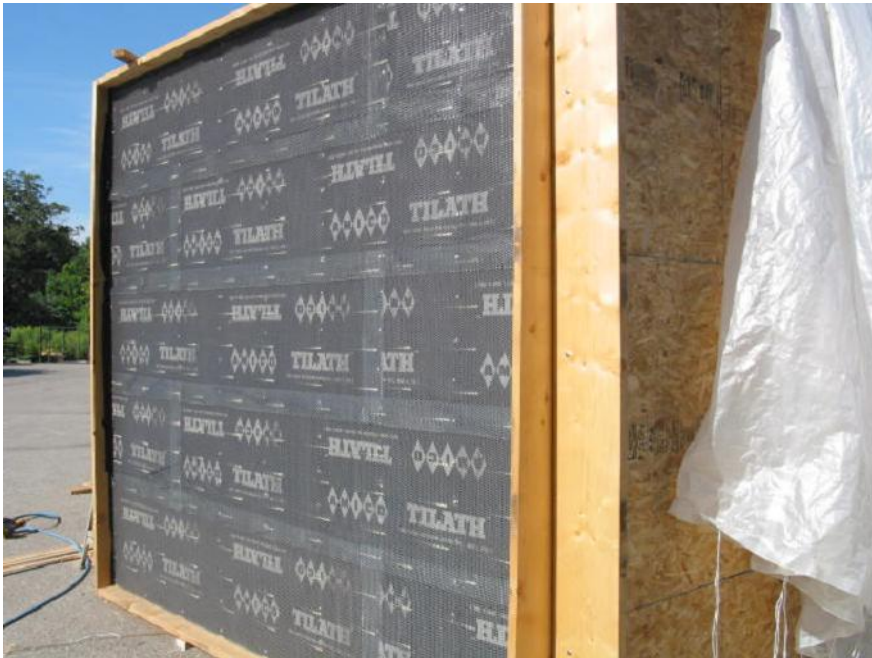
Photograph #3 – Completed application of paper backed lath
