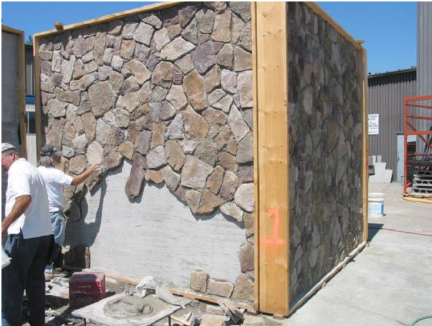
Photograph #5 – Application of manufactured stone
