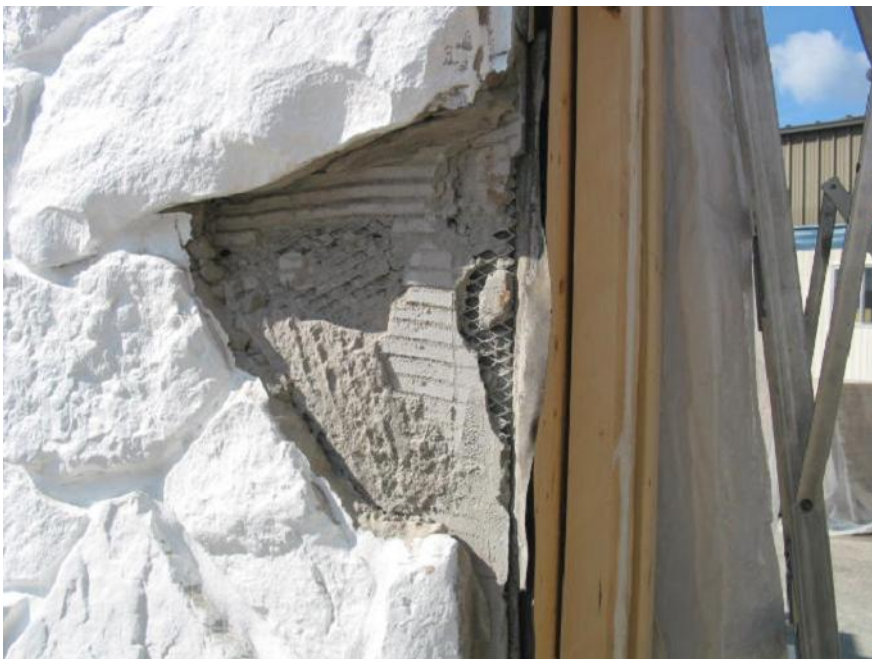
Photograph #8 – Typical failure of Panels #1 to #3
