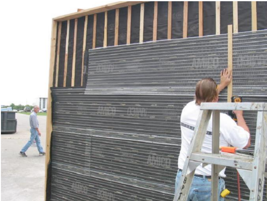
Photograph #2 – Paper backed lath being applied
