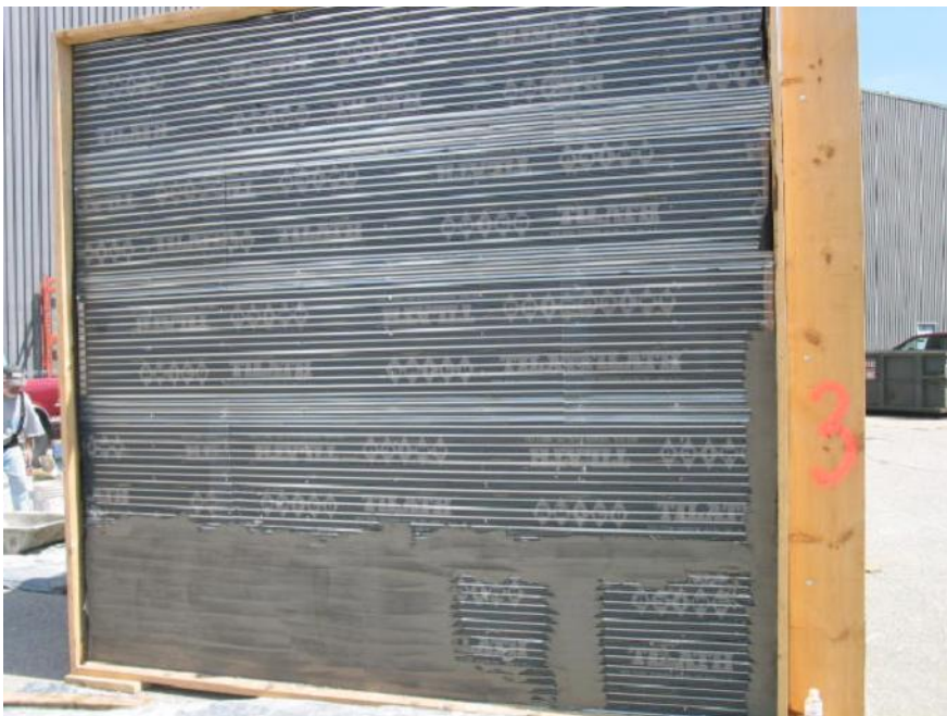
Photograph #4 – Start of scratch coat application of mortar
