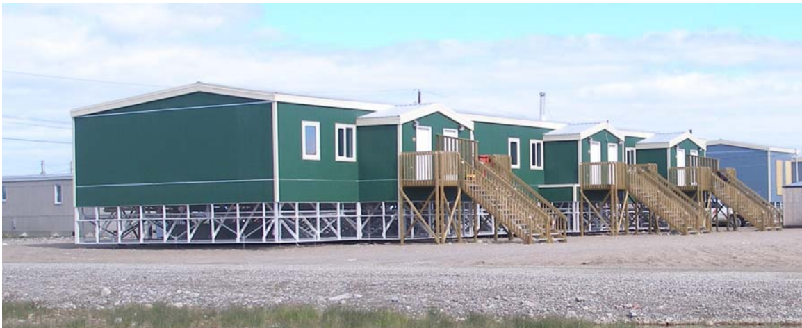
Figure 1: Completed NHC 5-Plex in Arviat, Nunavut
